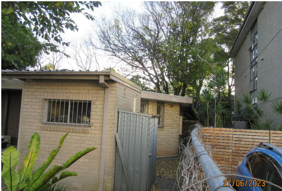
20 Rear of the building viewed from Allen Lane, adjacent to the northern site boundary.
